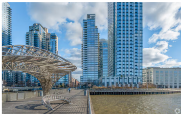
New condo buildings are rising
